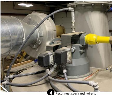
Route blower motor wiring through conduit and into disconnect panel.
