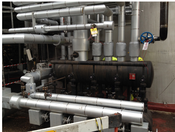
5EPT-312 condensate receiver package during
