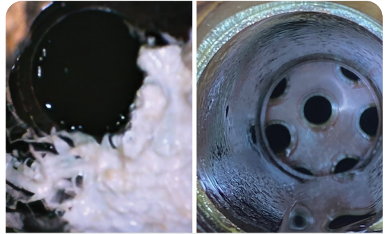
Heat exchanger tubes before and after continued use of nanobubble generator.
