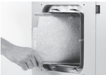
Step 1. Remove HumidiClean outer cover and remove tank access panel. Remove the old ionic bed inserts.
