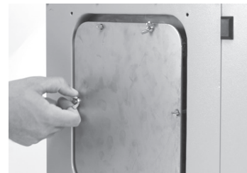
Step 3. Reinstall tank access panel and outer cover. Restart HumidiClean.
