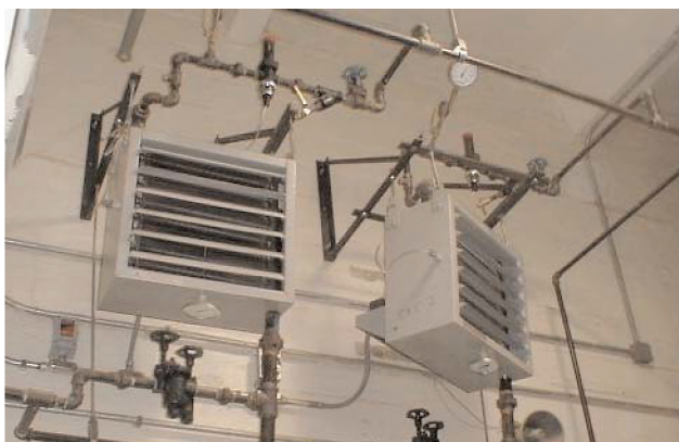
Armstrong Unit Heater Installation
